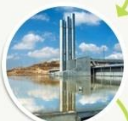
Organic Recovery Plant
