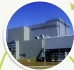
Energy Recovery Plant
